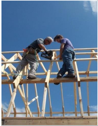
Figure 1.1 Installation of Batten which Requires Two Workers
