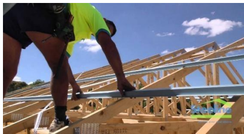
Figure 1.2 Dangerous Process Installation of The Battens
