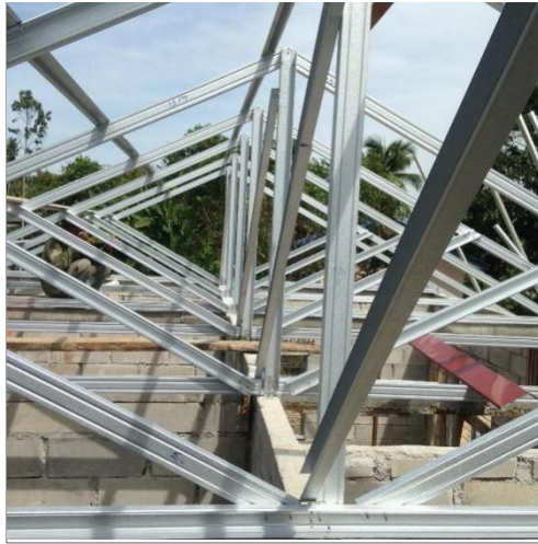
Figure 2.5 Figure of Complete Installation of Trusses.
