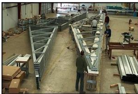
Figure 2.2 Prefabrication Process of Truss At Factory
