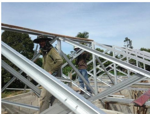
Figure 2.4 Assembling Process of Trusses
